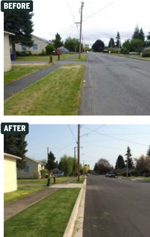
Figure 14. Local Residential Street Before and After SOS Rebuild
